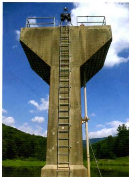
FIGURE 3: Hoisting inspection equipment onto riser structure
