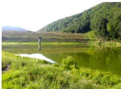
FIGURE 1: Hone Quarry Dam in Rockingham County
